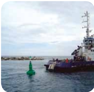
Sealite Poseidon Buoy installation, fitted up with an SLC310 light-head, Sint Maarten
